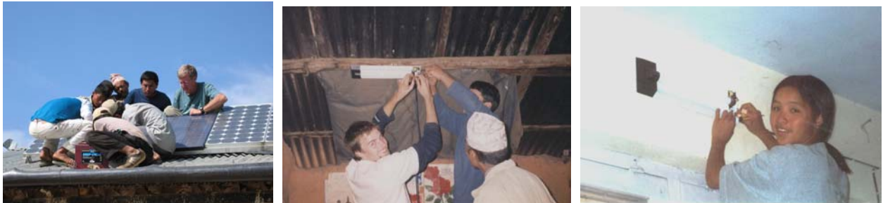
Solar Sisters volunteers installing Solar Home Systems
